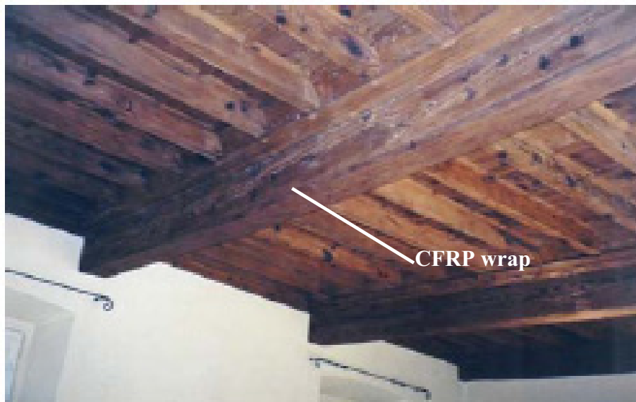
Figure 9-5 – Strengthening intervention on the main beam (Designers: ing. G. Ussia – Ardea Progetti & sistemi S.r.l.).
