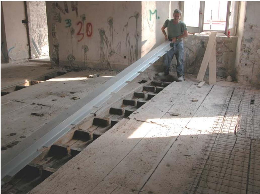
**Figure 9-4** –Strengthening intervention on the main beams (Designers: ingg. A. Giannantoni e F. Menghini, in collaboration with prof. A. Borri).
