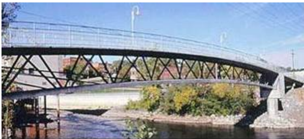
Figura 1-4 –Sherbrook Footbridge, Canada (1997). Luce: 60 m, resistenza a compressione: 200 MPa
