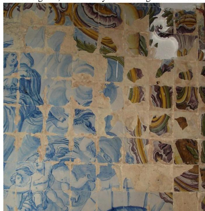
open spaces under the glaze resulting from delamination, causing a characteristic bubble that breaks away leaving a lacuna wherefrom the process of detachment later progresses. Cases are found nowadays where well over a third of the glazed surface has been lost [1] in a decay process that is in progression and will inevitably lead to the loss of whole panels of heritage value (Fig.3).
