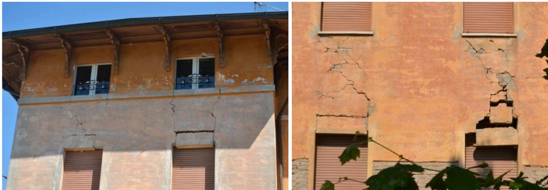
Fig. B-2 Damage in spandrels, with activation of both flexural and shear damage modes.
