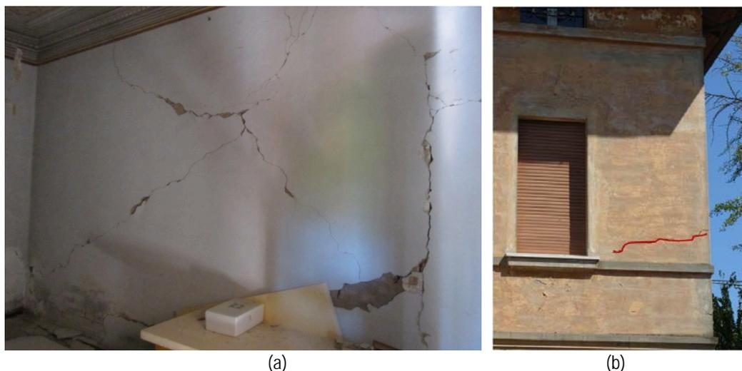
Fig. B -3 Cracks in piers: (a) shear failure in an inner wall; (b) flexural failure in a pier, located at the second floor of a perimeter wall, characterized by a low axial load.
