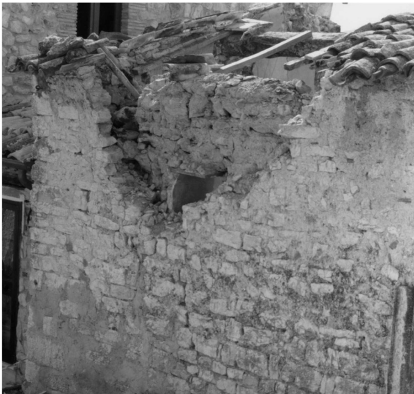
Figure 5-6 – Collapse due to horizontal bending.
