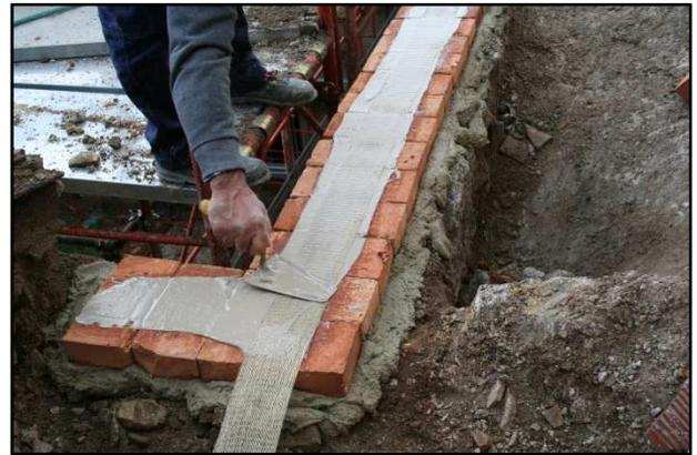
Figure 2.7 – Roof ring beams built with steel fabrics.
