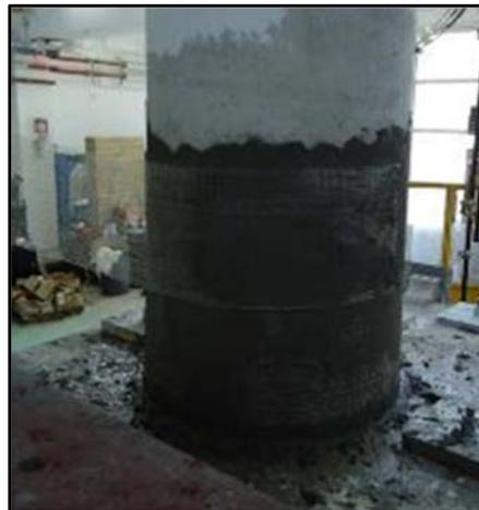
Figure 2.14 – Confinement of a column with unidirectional galvanized steel fibre strips and mortar.
