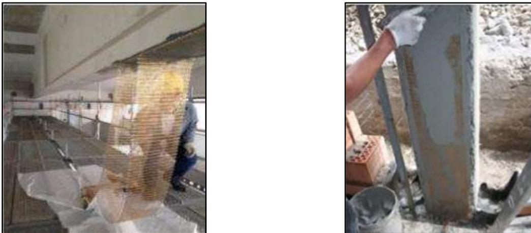
Figure 2.10 – Flexural strengthening of a beam and of a column with PBO fibre grid.
