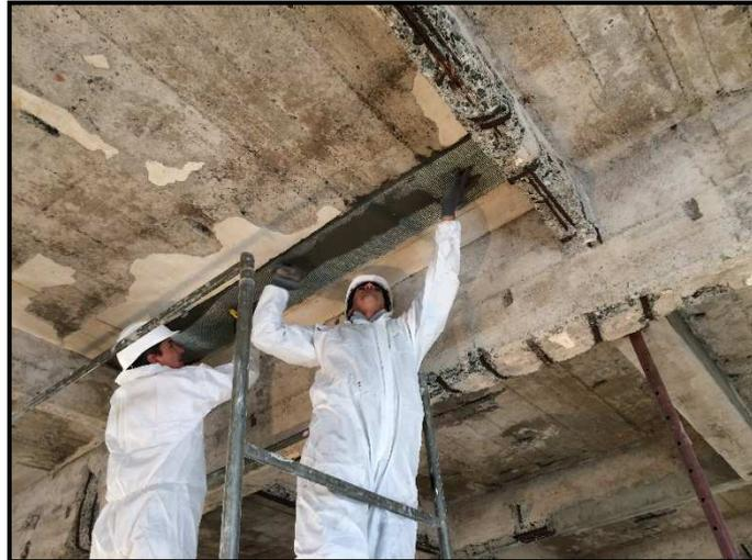
Figure 2.11 – Beam flexural strengthening with ultra-high strength unidirectional galvanized steel fibre strips and cementitious mortar.
