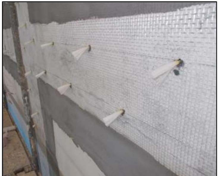
Figure 2.20 – Strengthening of walls against overturning with a FRCM system made of glass grid, mortar, adhesion promoter and glass fibre connectors.
