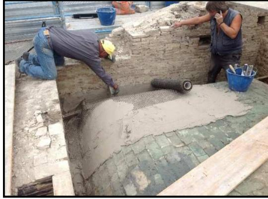
Figure 2.2 – Extradotal strengthening of a single-leaf vault with extensive application of basalt fibre grid and hydraulic lime mortar.
