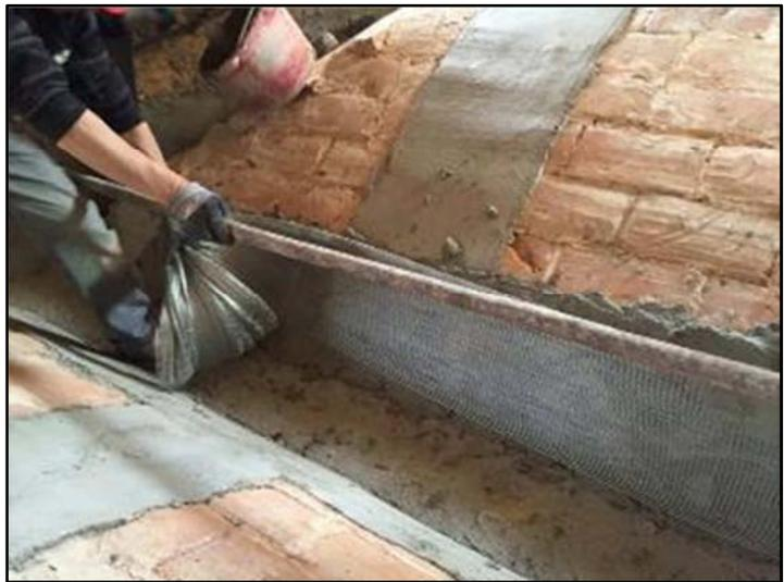
Figure 2.3 – Application of unidirectional galvanized steel fibre strips and mortar for the extradotal strengthening of masonry vaults.
