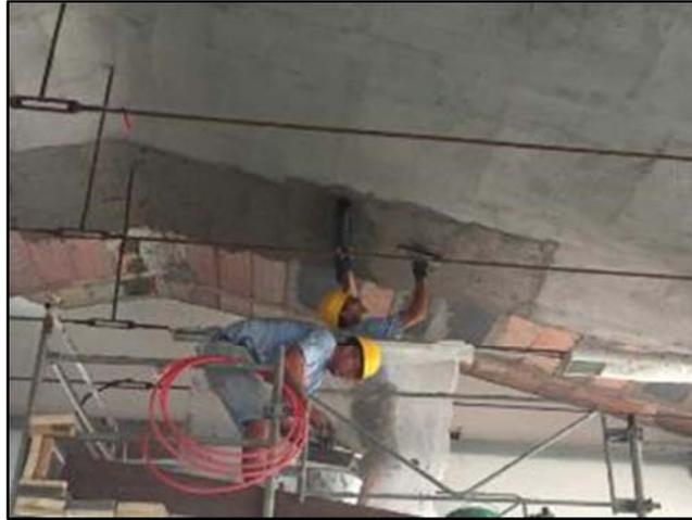
Figure 2.19 – Slab reinforcement (anti-detachment) with AR glass fibre grid and mortar.
