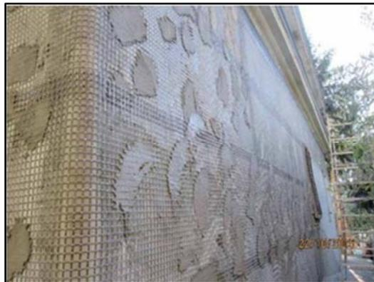
Figure 2.1 – Strengthening of masonry walls with basalt fibre grids.
