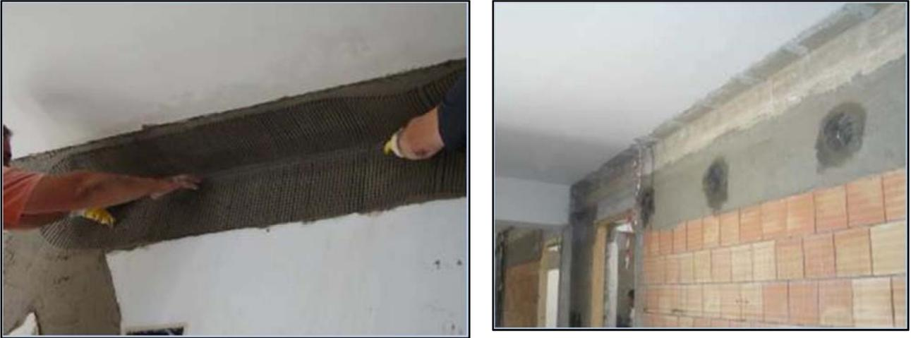
Figure 2.21 – Overturning protection of infill walls with different types of grids and anchors.
