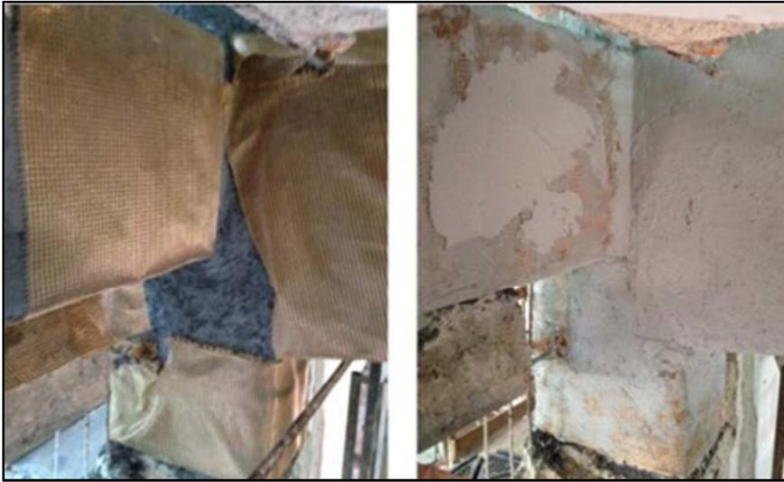
Figure 2.15 – Strengthening of beam-columns joints.
