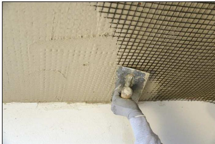
Figure 2.18 – Slab strengthening (anti-detachment).
