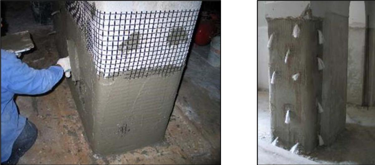
Figure 2.9 – Confinement of masonry column with AR glass fibre grid.
