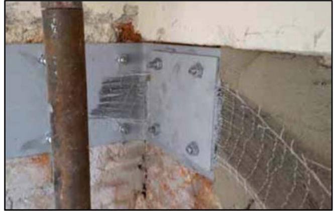
Figure 2.6 – Floor ring beams built with PBO and steel fabrics.
