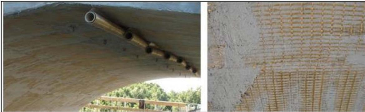
Figure 2.22 – Intradoxal strengthening of a concrete arch bridge with PBO grids.
