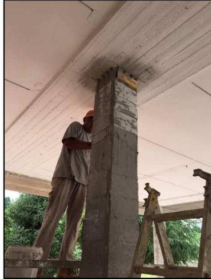
Figure 2.13 – Confinement of a column by means of ultra-high strength unidirectional galvanized steel fibre strips and cementitious mortar.
