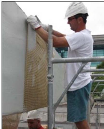
Figure 2.12 – Shear strengthening of a beam with PBO fibre grid.
