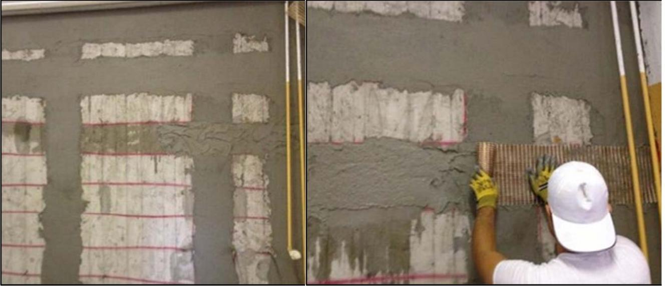
Figure 2.17 – Shear strengthening of reinforced concrete walls.
