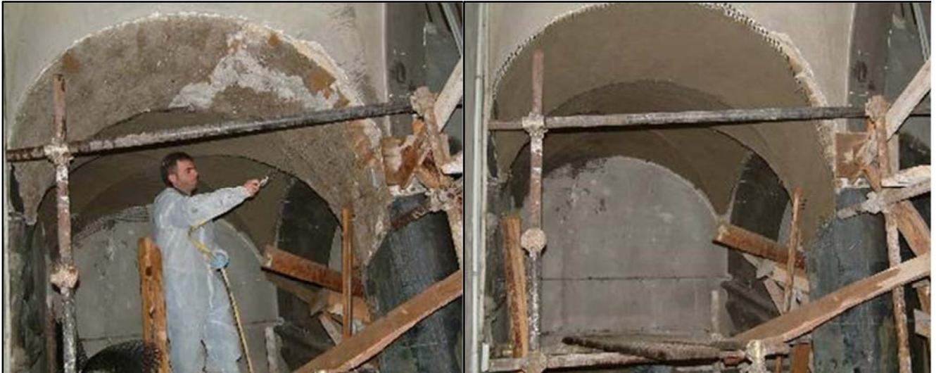
Figure 2.5 – Intradoxal strengthening of a masonry vault with AR glass fibre grid and mortar.
